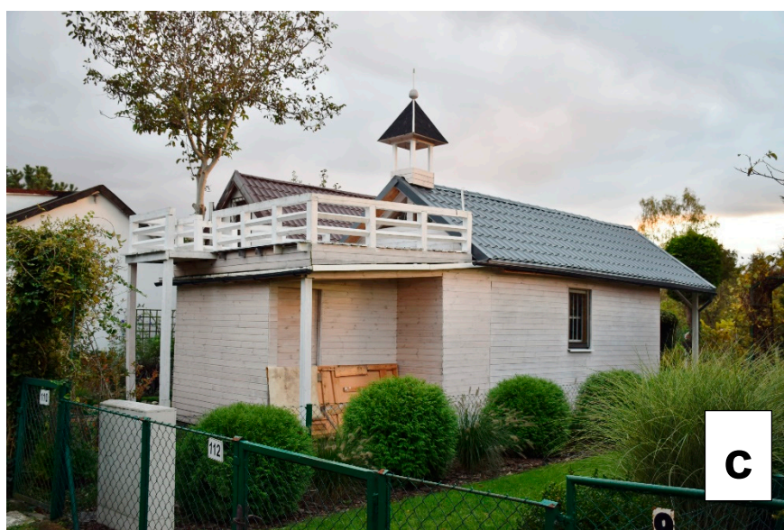
Figure 6. Examples of buildings inconsistent with applicable regulations, exceeding the permissible height (a,b), building material (a) and built-up area (c).
